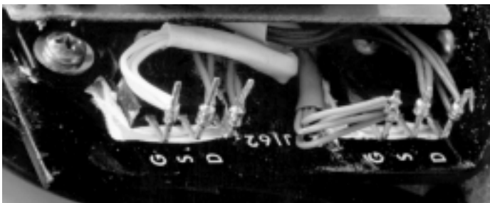
PHOTO 5: How the multiple wires of the Litz-type wiring are attached to the MOSFET leads.
