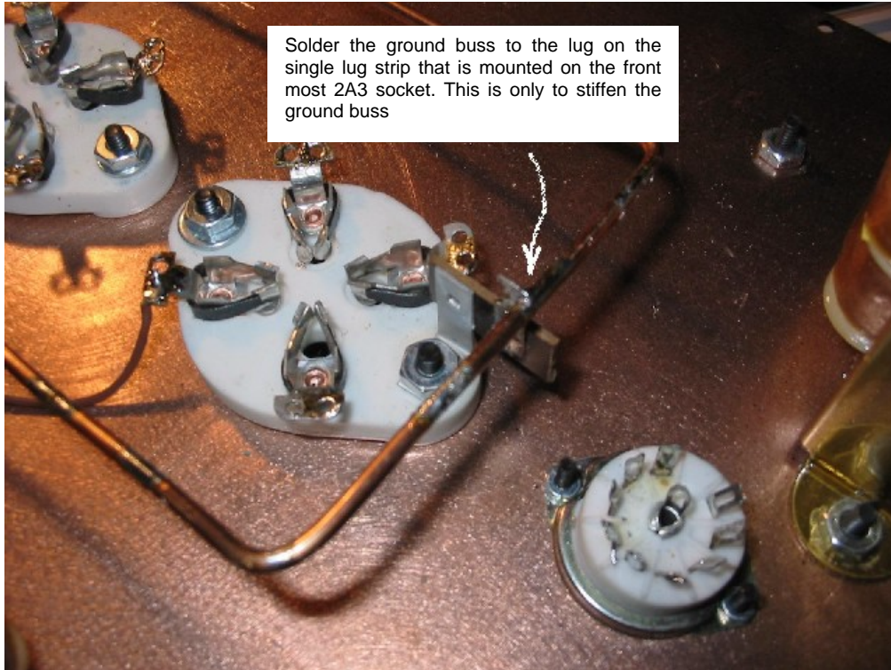
Figure 21. Detail of the ground buss connection to the stiffening solder lug.
